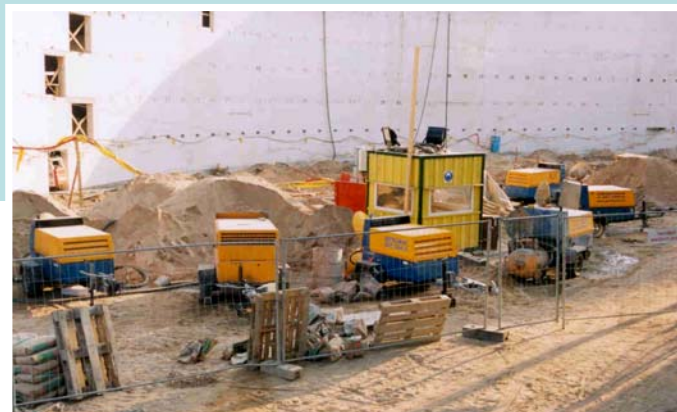
Large-scale building site with UELZENER ESTROMAT screed machines
